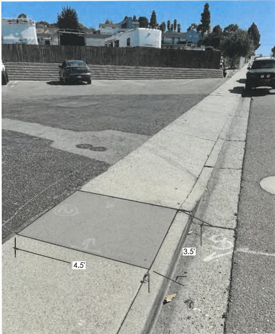
16 SF OF SIDEWALK PANEL REPLACEMENT PER CITY STANDARD 4110
