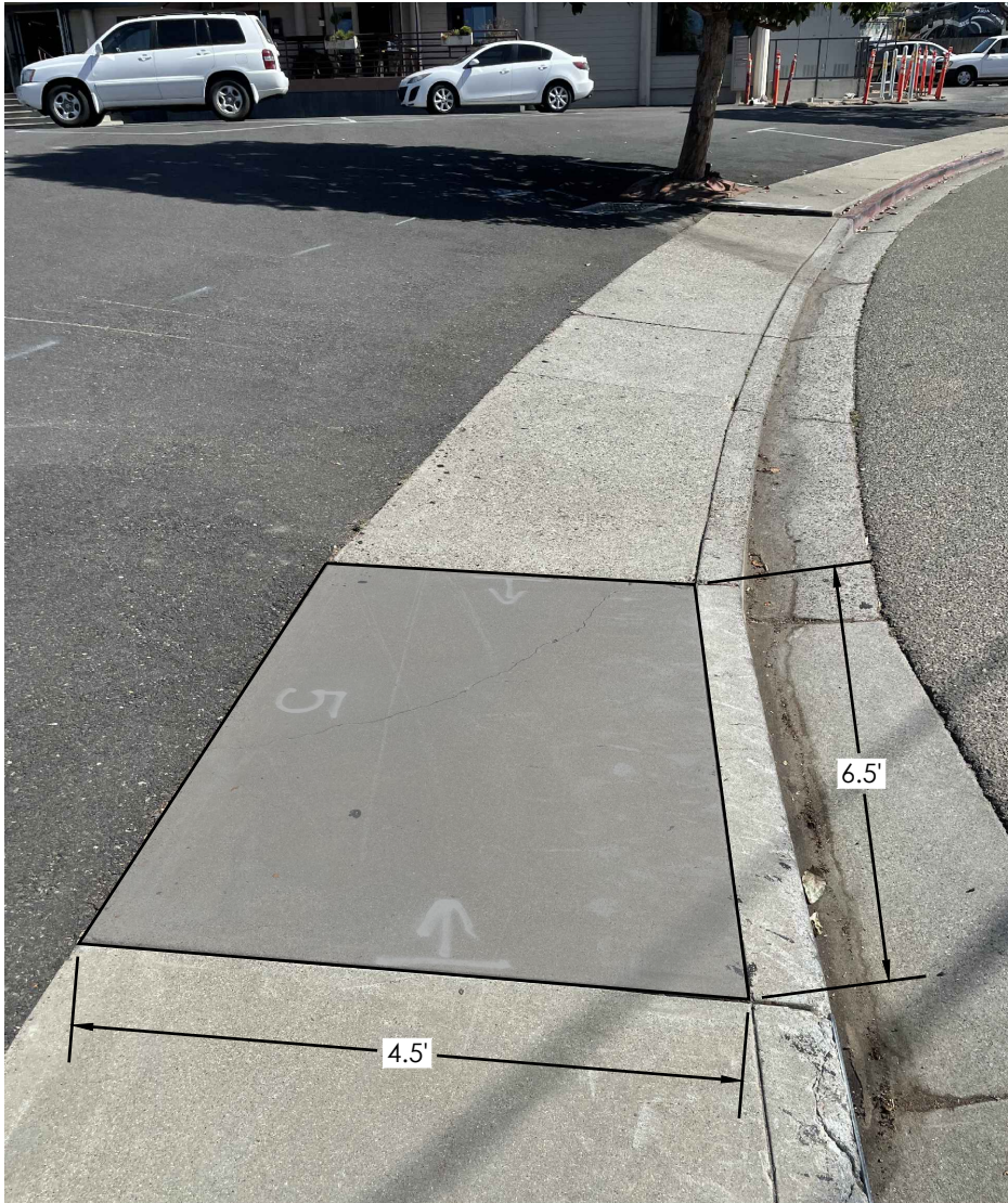
29 SF OF SIDEWALK PANEL REPLACEMENT PER CITY STANDARD 4110
