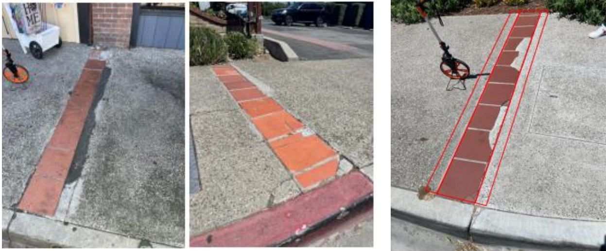
1242 (LF) Existing Tile Bands
