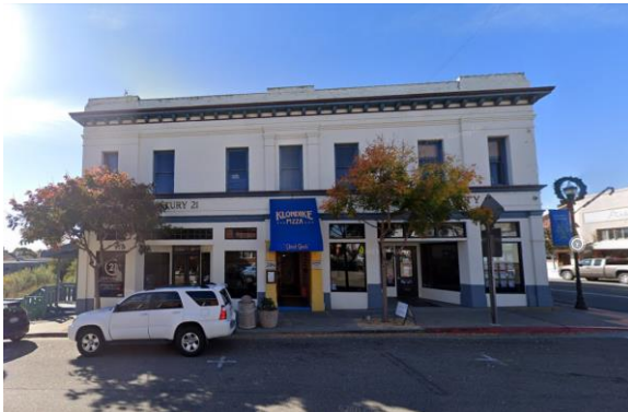
Figure 2. The northeast façade, facing Bridge Street. Source: Google Street View, 2020.
