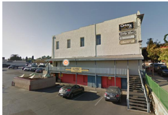
Figure 5. The southeast facade. Source: Google Street View, 2018.
