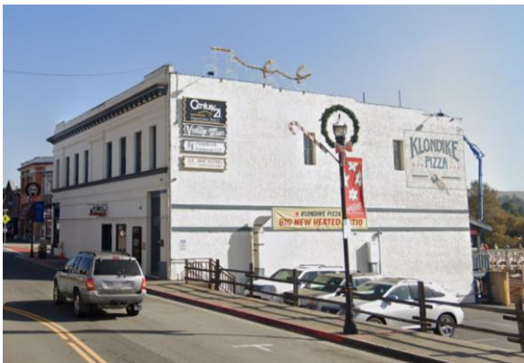
Figure 4. The southwest facade. Source: Google Street View, 2020.
