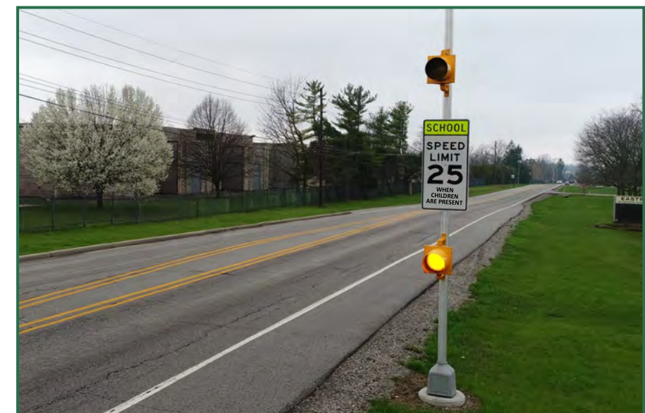
School Zone Speed Limit Sign with Flashing Beacons
