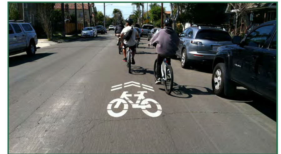
Shared Lane Marking
