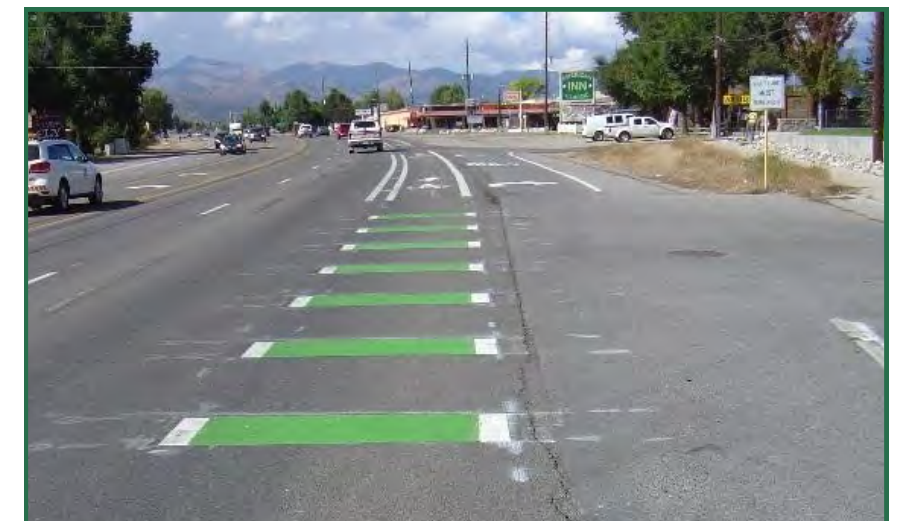
Green Colored Pavement for Bike Lane in Merge Area
