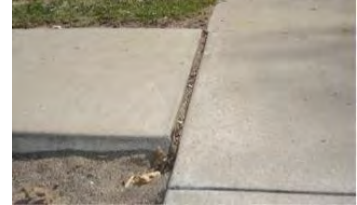
Openings in the surface of an accessible route may not be large enough to admit a \frac{1}{2} " dowel.
