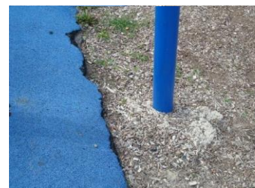
Surfaces should drain properly to prevent hazardous conditions caused by erosion and other forces. In the photo on the right, erosion has broken down the surfacing and exposed concrete footings.
