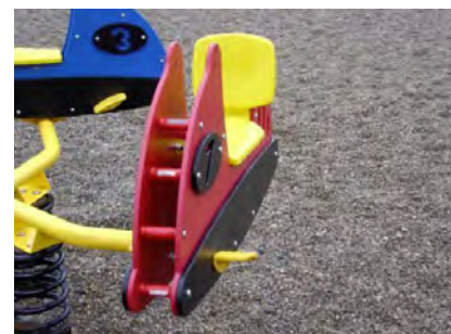
This spring rider is missing a handhold. This missing part is a danger to users.
