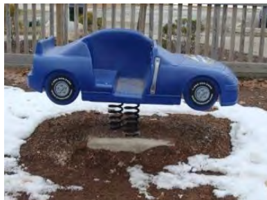
The concrete footing is exposed.
