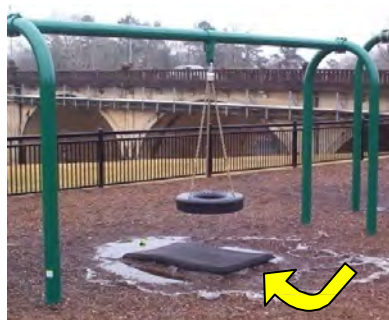
The concrete edge of this wear mat is exposed.
