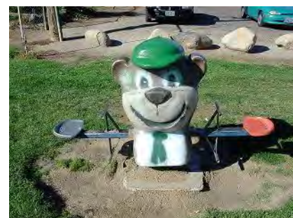
In addition to having unacceptable surfacing around it, this seesaw's exposed concrete footing poses a hazard to children.
