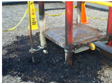
Fire damage to this playground surface has made it unsafe.
