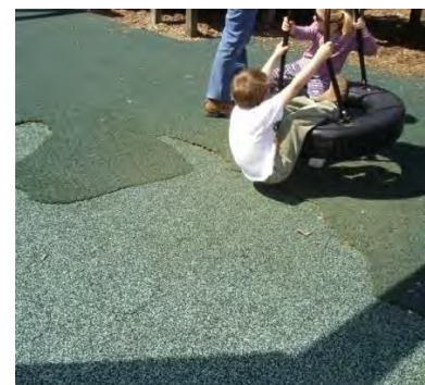
This poured-in-place surfacing requires repairs.
