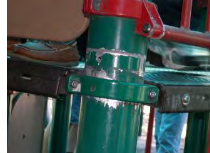
This collar has become loose and the deck is slipping. Report such loose hardware and prevent children from playing on the deck.
