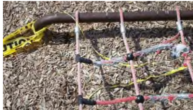
Worn ropes and an exposed anchoring device make this component unsafe.
