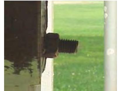
More than 2 threads are showing, so this bolt is a hazard.
