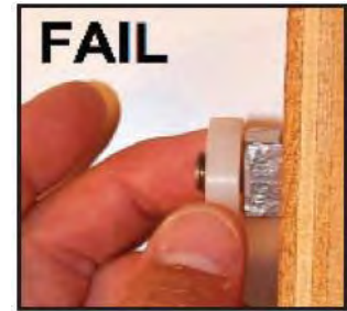
Source: CPSC This bolt end is an unsafe protrusion.
