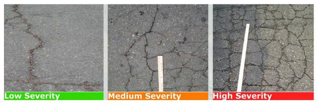
Image 1: Alligator Cracking
