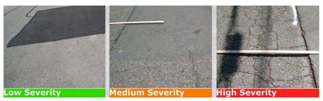
Image 5: Patching and Utility Cut Patching
