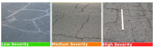
Image 2: Block Cracking
