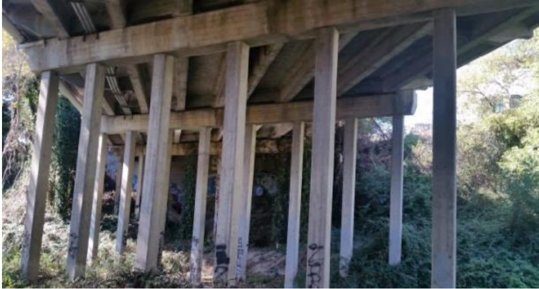
Figure 1: Traffic Way Bridge Piles
