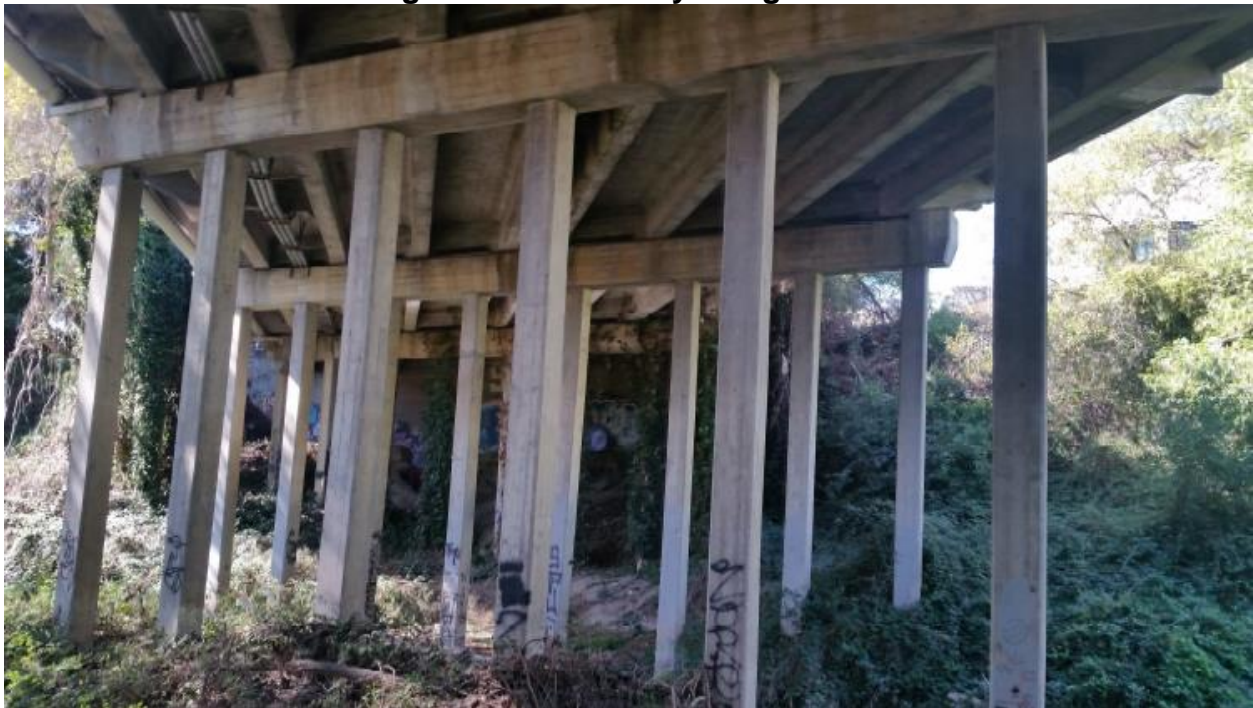
Figure 1: Traffic Way Bridge Piles
